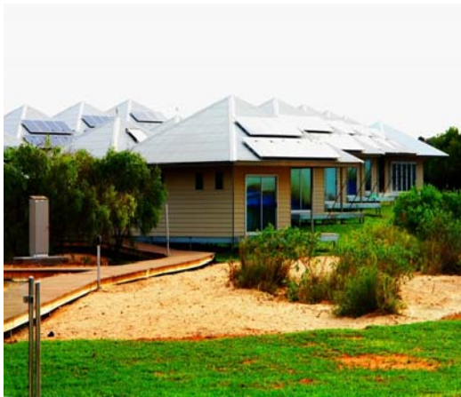
Figure 9a: Eco resort villas with photovoltaic panel installation.
