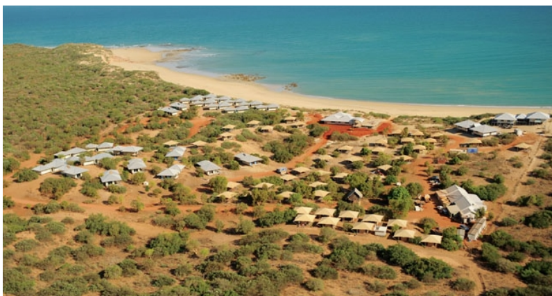
Figure 7: Aerial view of the Eco Beach Resort
