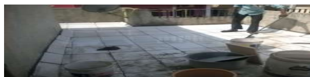
Figure 8: Building photographs after applying insulator - Tiles at Roof and Wall
