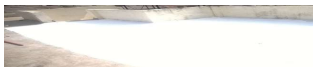
Figure 7: Building photographs after applying insulator - Lime at roof
