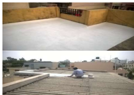
Figure 6: Building photographs after applying insulator - SRP at Roofs
